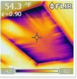
Air Leakage at Attic Hatch: The infrared camera suggests a poorly sealed and uninsulated attic hatch. The outside air from the attic space is leaking into the living space and making the upstairs hallway extremely cold. Since this is where the thermostat is located, the furnace runs more frequently than it needs to in order to maintain a consistent temperature.
