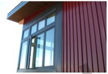
Metal window frames conduct heat at 1000 times the rate of wood, vinyl or fiberglass. Triple pane fiberglass windows like those in the picture on the right conduct very little heat, seal tightly, and have an insulating value that's better than most insulated walls!
