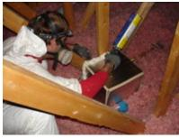
Can lights are a huge source of energy loss in an attic. Unfortunately, you can't just caulk them up and blow insulation over them. It's important to build a "top hat" around the can light with rigid foam and then seal it together with spray foam. This keeps the light from overheating while preventing significant air leakage through the light into the attic.
