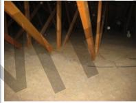
This attic has very little insulation and none in some cases. By installing 10 to 15 inches of insulation in the attic, you can save a significant amount of energy. When doing so, it's really important to first clean out the existing insulation and then sealing all of the penetrations and cracks in the attic floor that's
