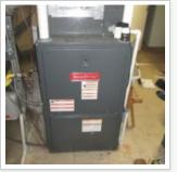
Congratulations! You have a modern high efficiency furnace. This system is a sealed combustion unit. That means that any flue gasses produced by burning the natural gas go directly outside without the opportunity to leak into your home. Also, fresh air from the outside is brought directly to the burners in the furnace as opposed to pulling air from the house. This keeps the cold outside air in a closed loop and keeps the exhaust air outside where it belongs!
